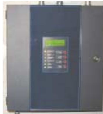
(Fig. 6.3) Control panel with alphanumeric annunciation display.
