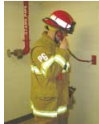
(Fig. 6.8b) A firefighter using a handset in a remote jack located inside a stairway.
