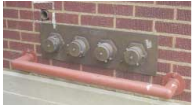
(Fig. 5.3) A 4-inlet FDC. It would probably be more efficient, and give the fire department more options, to have placed two, 2-inlet FDCs in different locations on this building.
