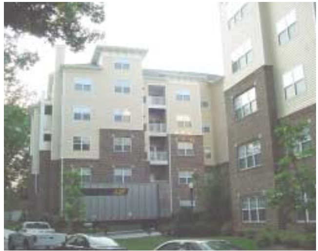
(Fig. 3.6) This building has six occupied levels from this view. However, it is classified as a four-story building by the code that was in effect during its construction. As such, an NFPA 13R residential sprinkler system (with no sprinklers in the combustible attic or in the floor/ceiling assemblies) protects it.
