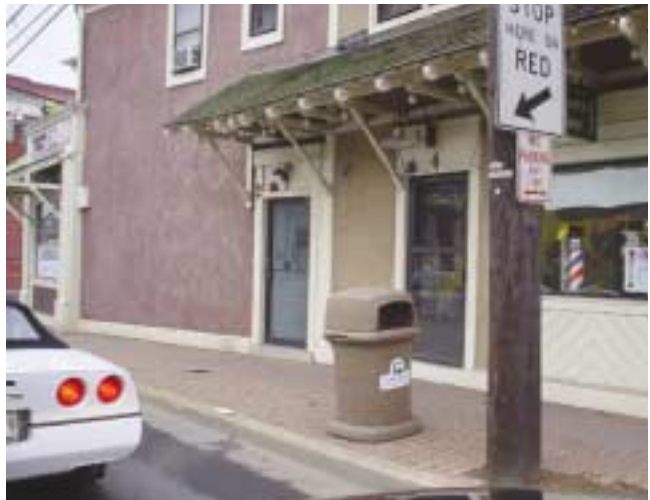
(Fig. 6.6) Strobes above each tenant entry door indicate the tenant where an alarm originates in this building, which has multiple tenants with different addresses fronting on two streets.
