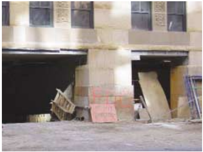
(Fig. 5.15) A temporary FDC labeled with a large colorful sign, as well as large letters "FDC" spray-painted on the building.
