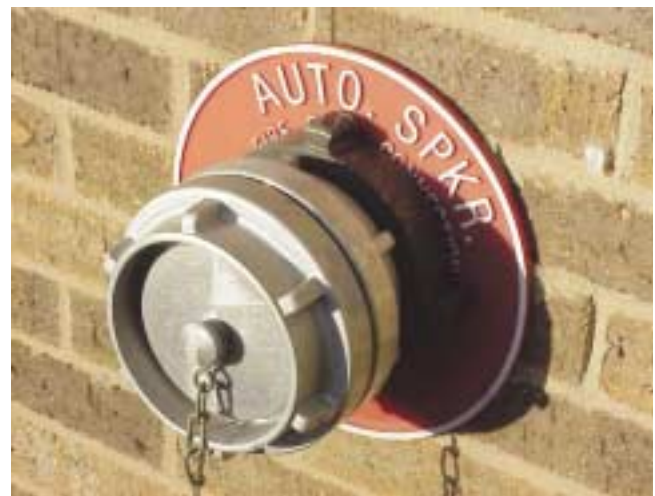
(Fig. 5.4) A quick-connect type of FDC.
