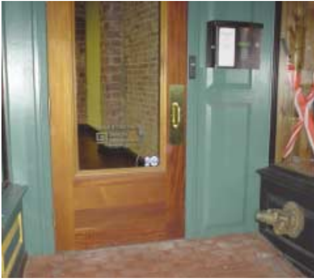
(Fig. 5.9) An FDC pointed directly across the main entrance of a restaurant. A connected and charged hose line would impede both egress and entry.
