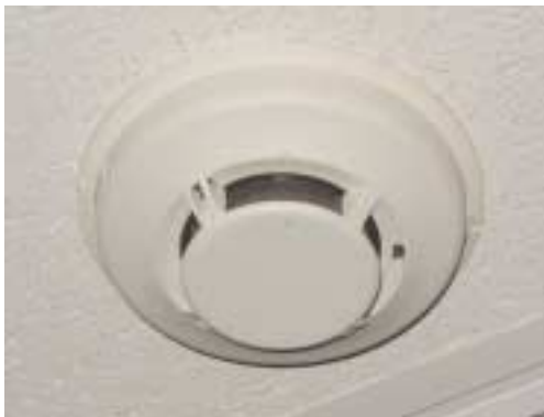
(Fig. 6.1a) Initiating device (smoke detector).
