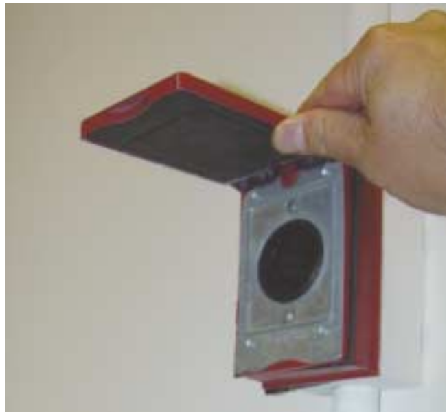
(Fig. 7.2) A weather-resistant receptacle cover opened, showing the twist-lock receptacle.
