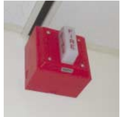
(Fig. 6.1c) Notification device (horn/strobe).
