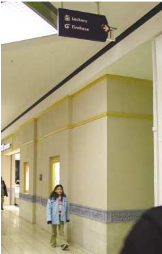
(Fig. 4.8) Sign to identify hose connection location in a shopping mall.
