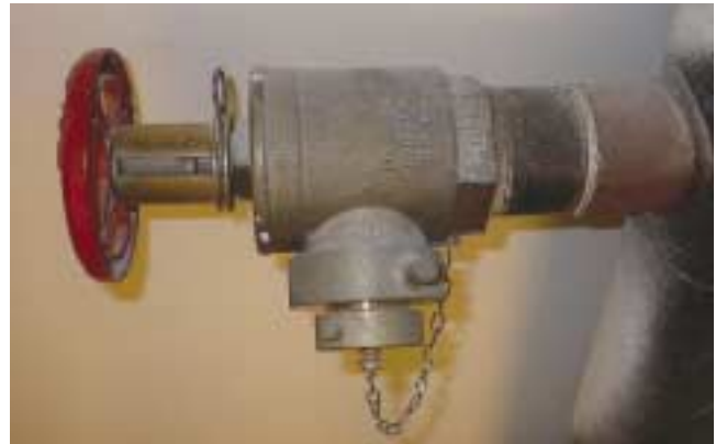
(Fig. 4.10) Hose connection equipped with a pressure regulating device.
